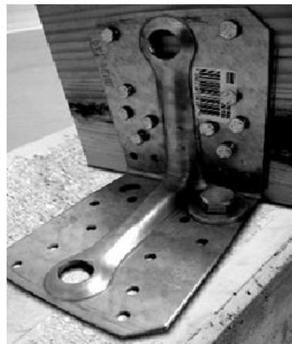
**Fig. 8.** Example of the fixing of carpentry joints in the timber – concrete combination – the proper placement of the nails and bolts [8]
