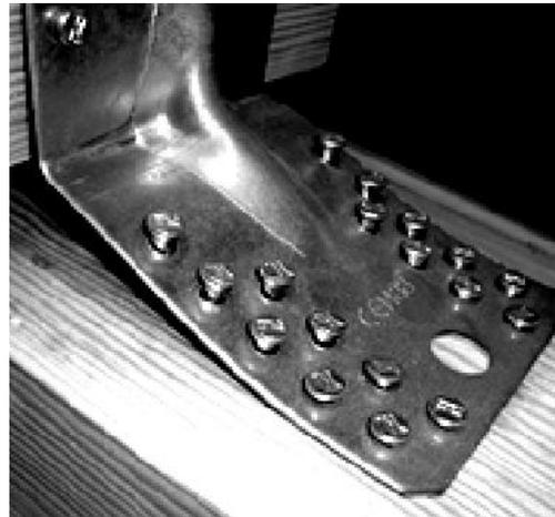
**Fig. 7.** Example of the fixing of carpentry joints in the timber – timber combination – the failure because of too large distance of the nails to the break line [8]
