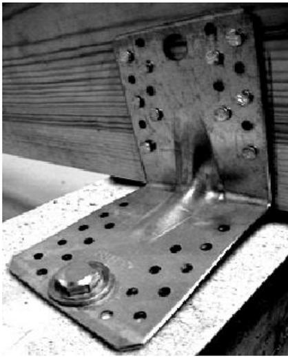
Fig. 9. Example of fixing of carpentry joints, a timber – concrete combination – the failure because of too large distance of a bolt to the break line [8]
